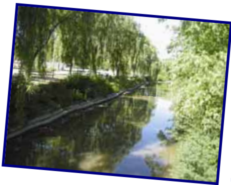
Streambank stabilization at Ford Field in Dearborn
